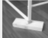
Wood block to pro- tect the floor
