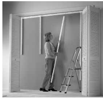
Hook the Hang Standards on the HangTrack.
