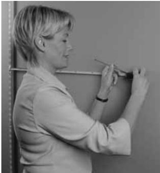
**Step 5** Prepare for the second wallband by measuring and mark the c/c-distance, not more than 900 mm between the wallbands. Place a bracket in the second wallband on the same height as the first one. Be sure of placing the wallbands parallel with one another and to place the both brackets in the same height.
