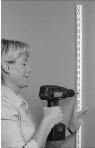
**Step 1** Install the first wallband at desired height on the wall. Start by drilling a hole in the wall for the second hole (from the top) in the wallband. Fasten with one screw.
