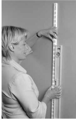
**Step 2** Check with a level that the wallband is hanging in vertical position.
