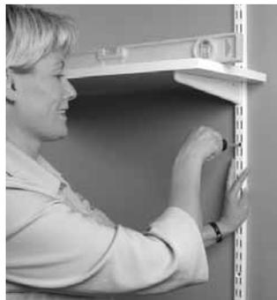
**Step 6** Place a shelf on the brackets and check with a level that brackets are in level. Drill holes and fix the wallband with screws.
