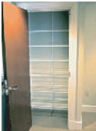
Faculty storage closet
